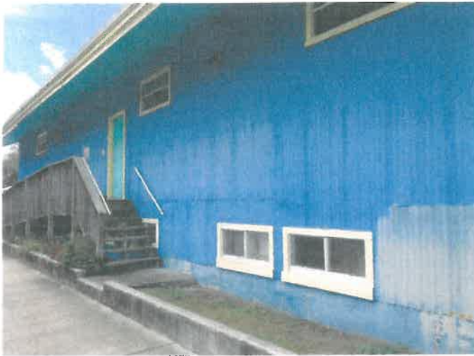
1. Street facing side of the Building
