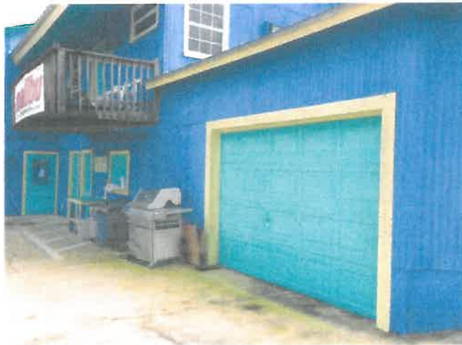
3. Back/Lake facing side
