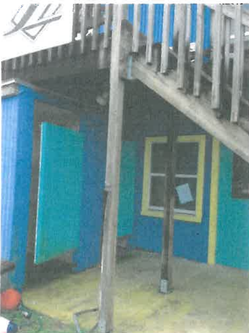
7. Back/Lake side of Building (remove current showers)
