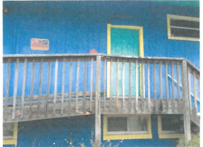
2. Street facing side of the Building
