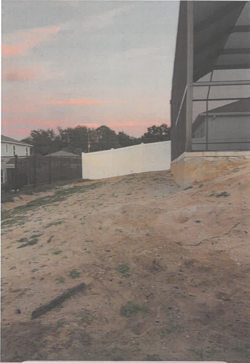
Photo 8. Back of the pool/property before plants and turf installation.
