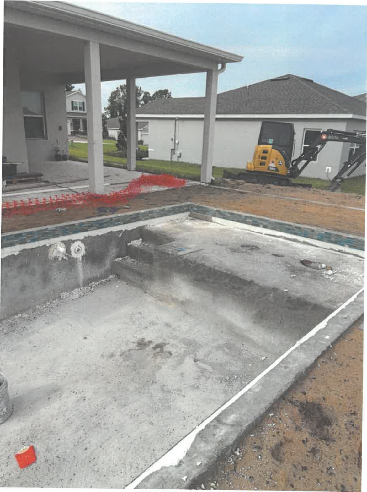
Photo 7. Pool in construction showing side slope
