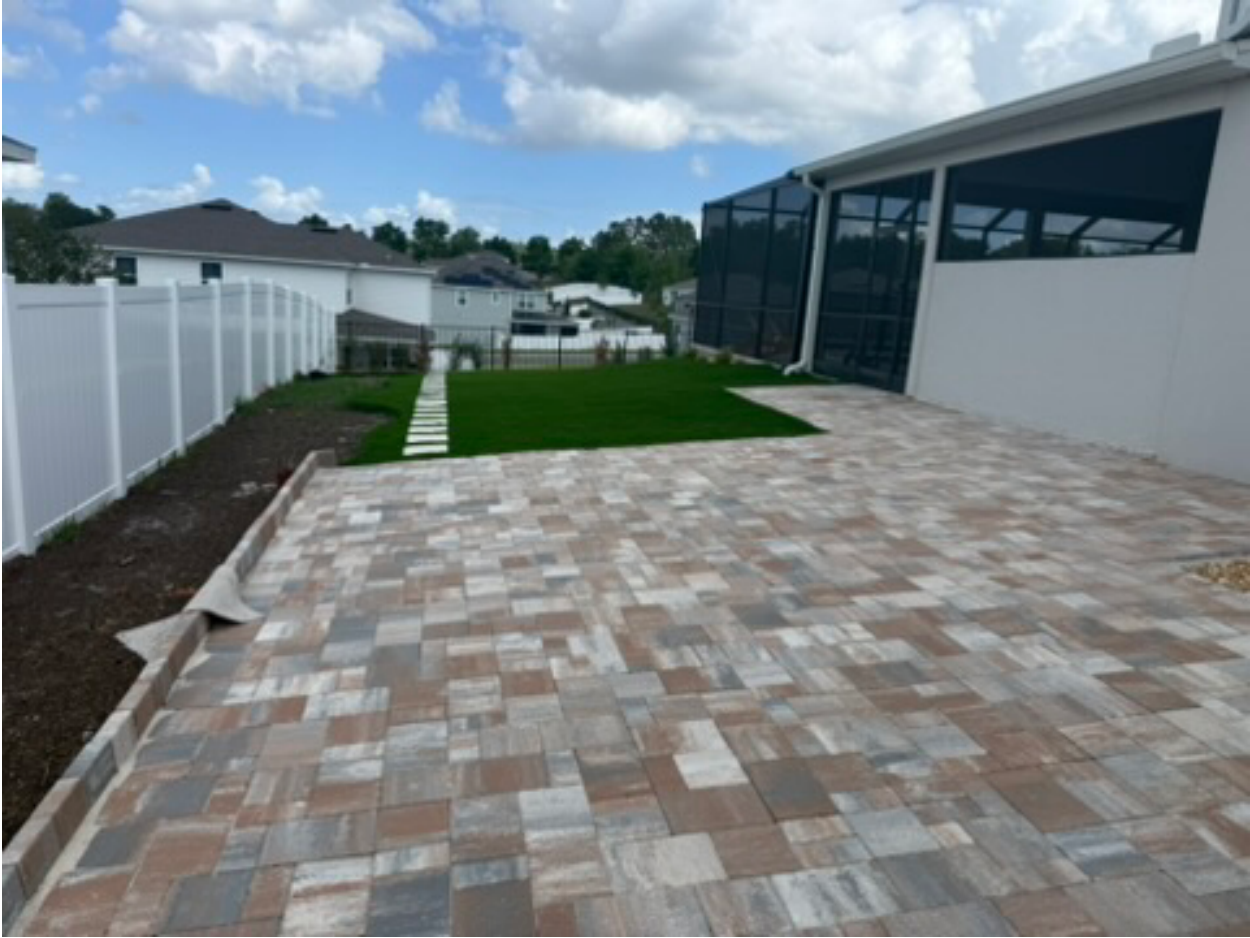
Figure 1: West Property Line Looking North
