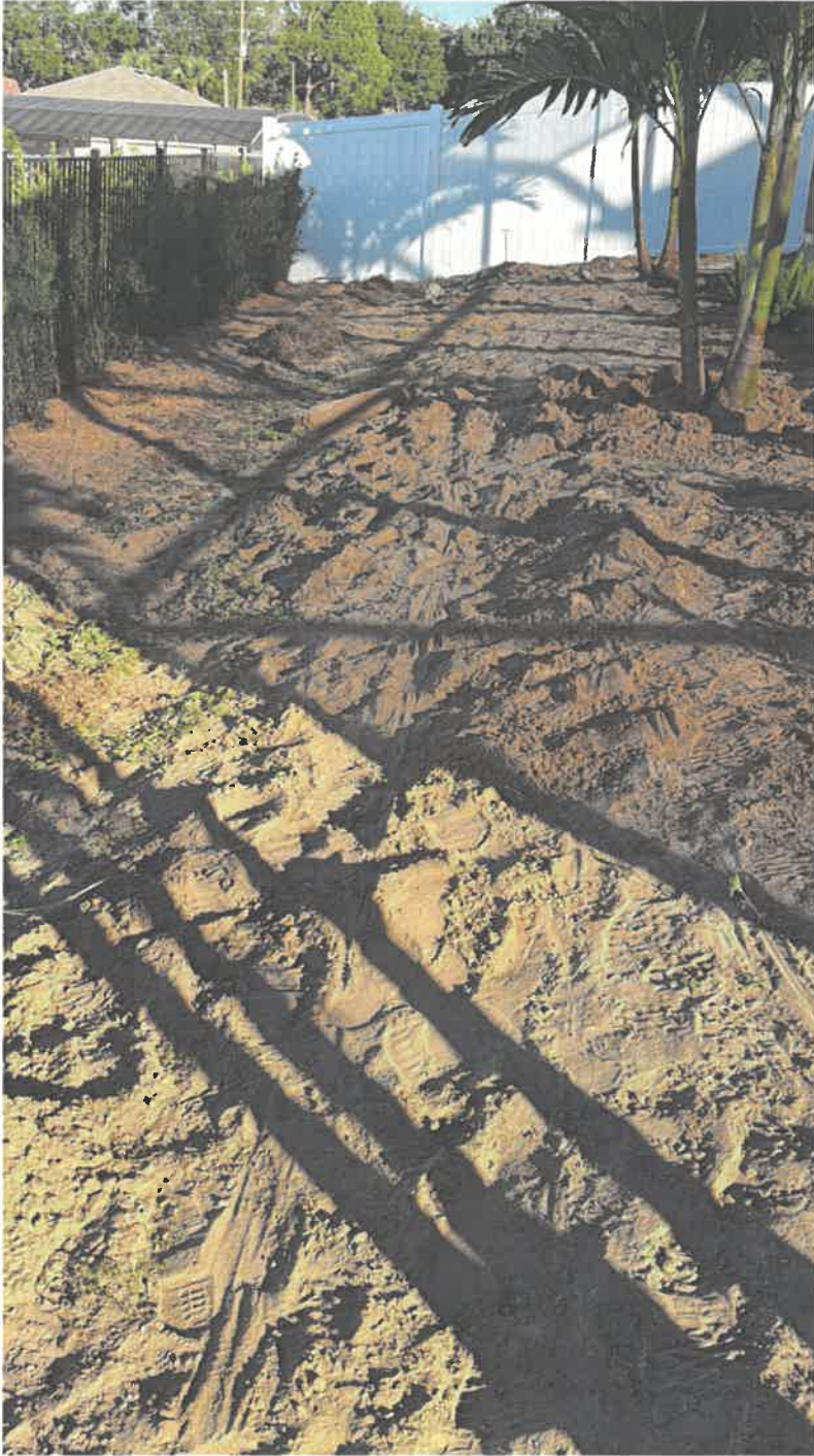
Photo 9. Back side of the pool/property during plants and turf installation.
