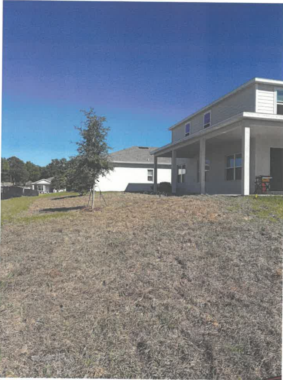
Photo 1. Backyard and lanai before gutter installation
