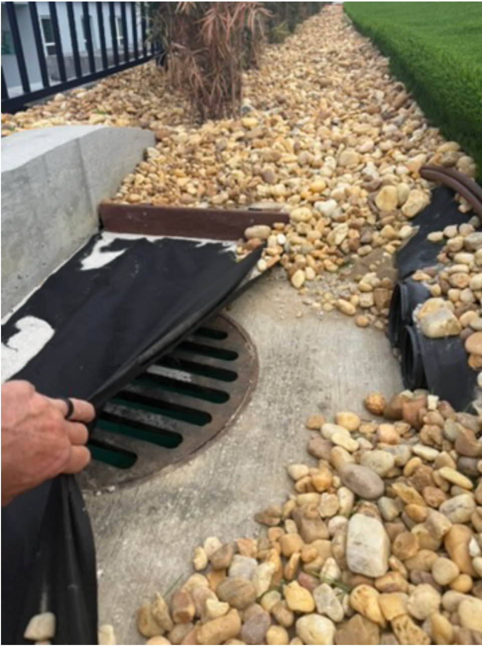
Figure 4 – Area Drain At Rear Property Line
