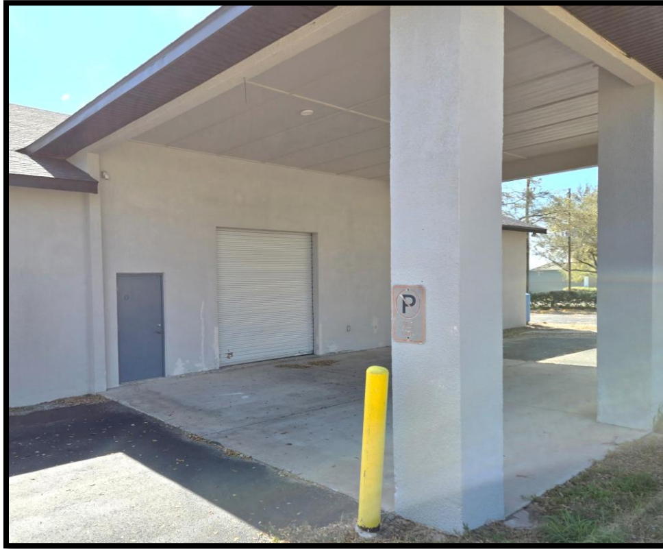
North side of building with large roll up door
