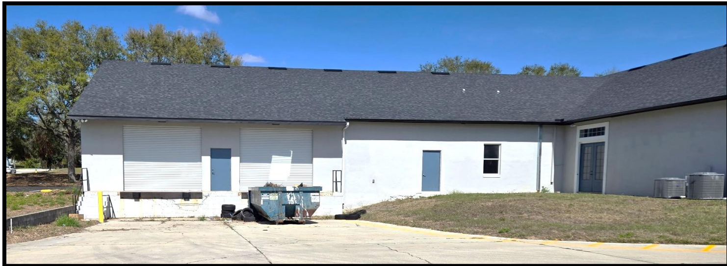
South side of building with large roll up doors and loading dock
