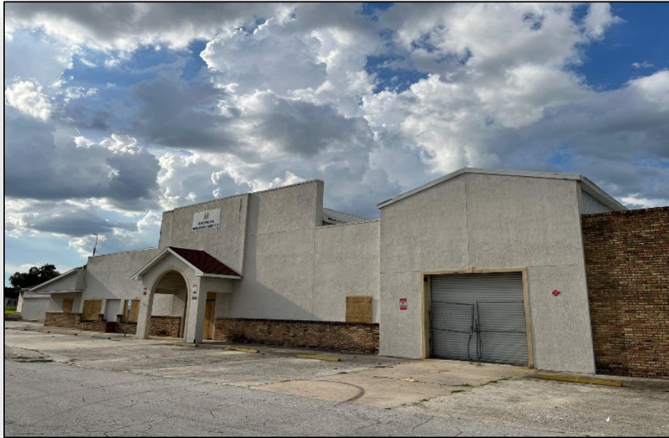
Figure 12 – Photo of lumberyard building to be demolished, 1000 Carroll Street (LA05472).
