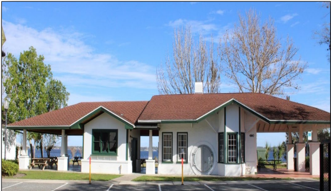
Figure 105 – The Clermont Railroad Depot (LA05645) built in 1925.
