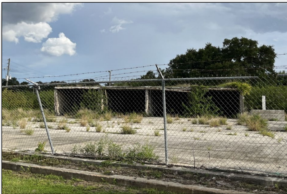
Figure 13 – Building in process of demolition, 1111 Carroll Street (LA05474).
