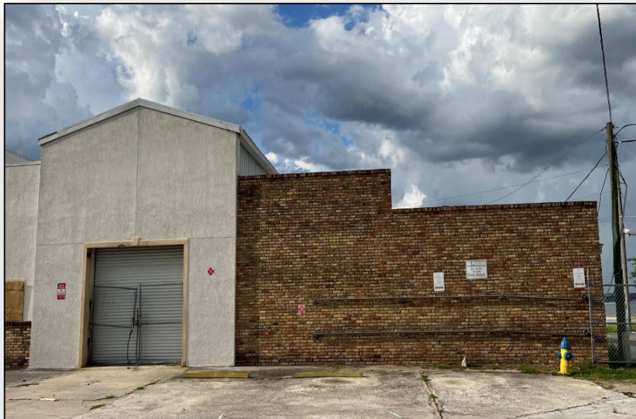
Figure 119 – 1000 Carroll Street (LA05472), brick and stucco detail.
