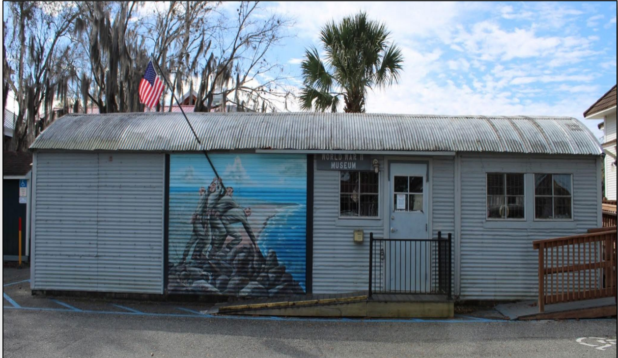
Figure 106 – The Quonset Hut (LA05646), built in 1943.
