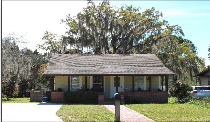
Figure 69 – 555 W. Desoto Street (LA05480) Frame Vernacular, Hall and Parlor
