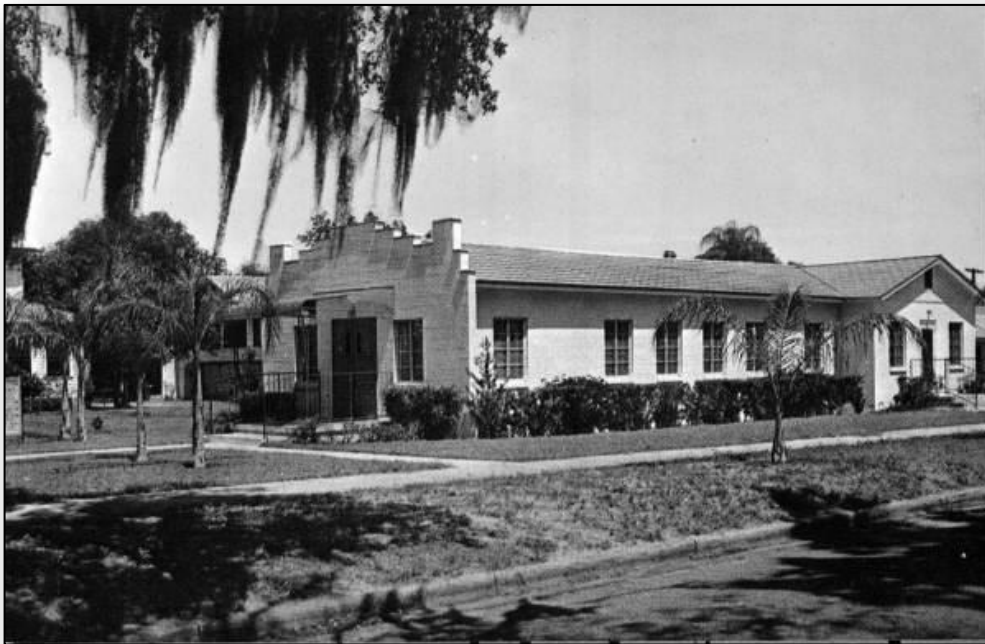
Figure 66 – The original First Church of Christ, Scientist building; it would be substantially remodeled in 1970. (Source: Florida Memory, http://www.floridamemory.com/items/show/138792 .)
