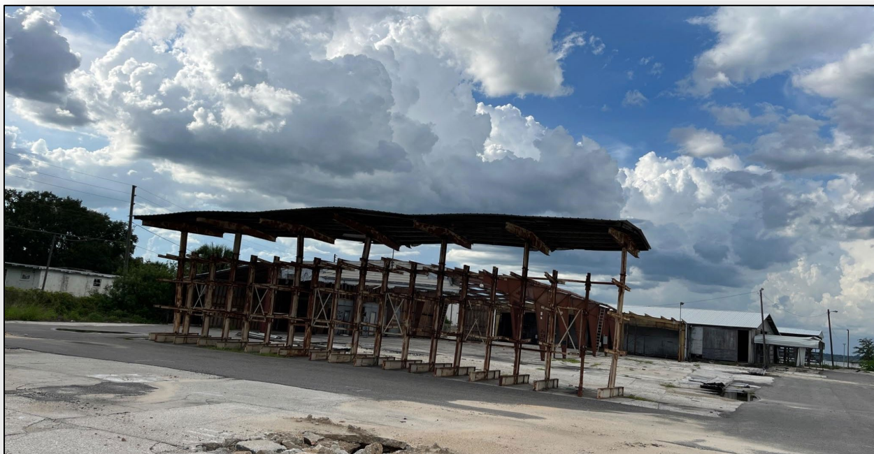
Figure 125 – Structure associated with lumberyard use, facing south.
