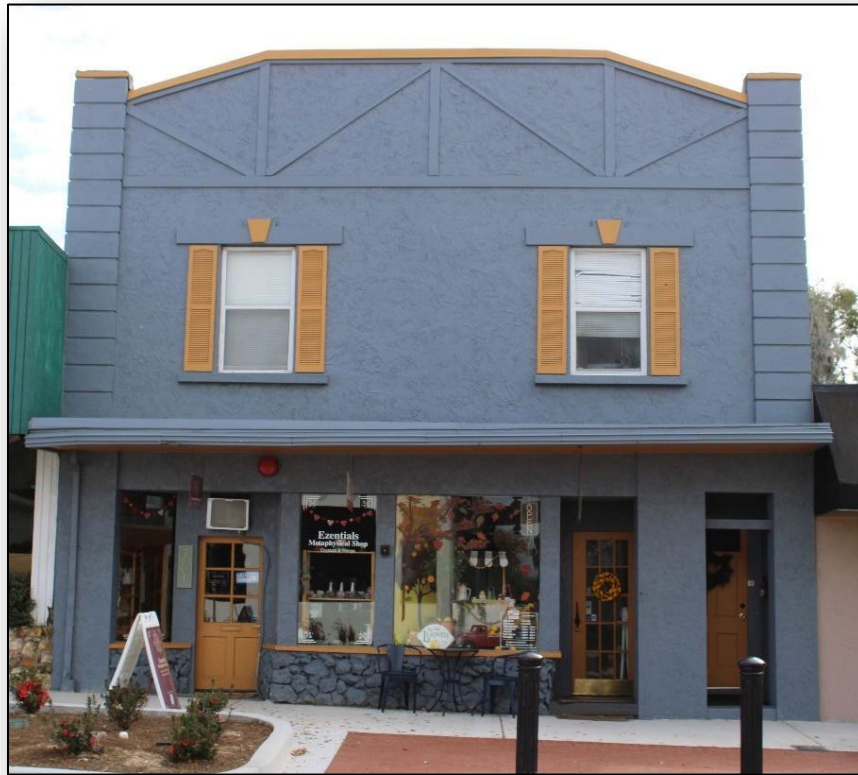
Figure 81 – 761 W. Montrose Street (LA05590) Two-Part Commercial
