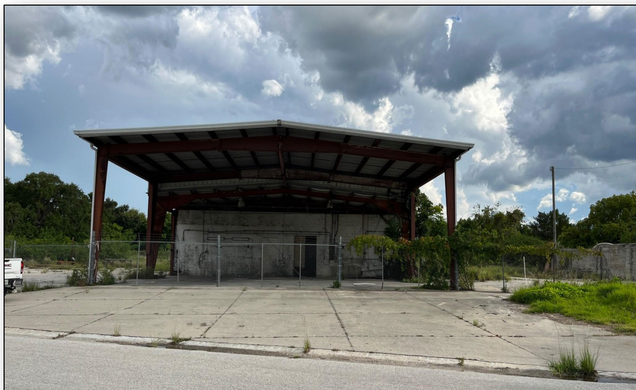
Figure 129 – Structure associated with lumberyard use, facing south.
