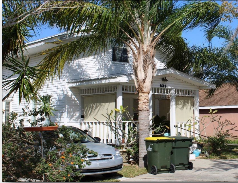
Figure 73 – 838 W. Montrose Street (LA05608) Frame Vernacular
