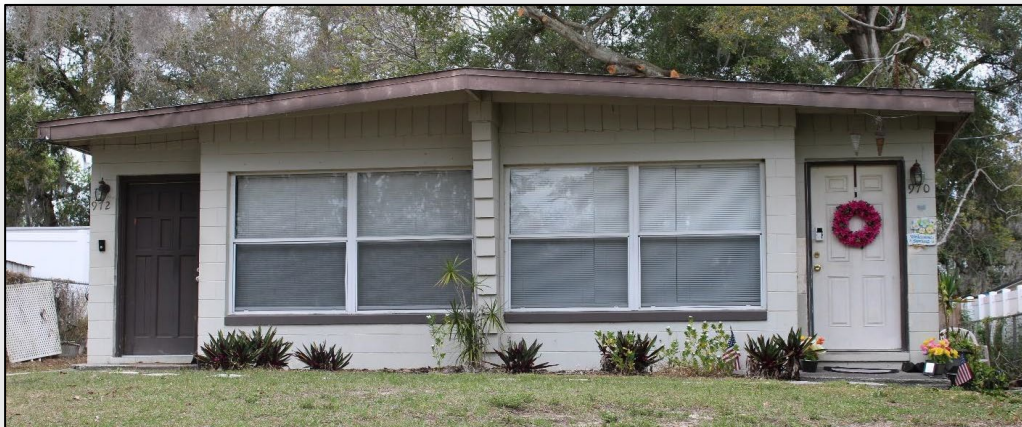
Figure 75 – 970 W. Juniata Street (LA05520) Masonry Vernacular
