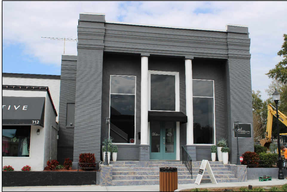
Figure 90 – 702 W. Montrose Street (LA03998) Neoclassical Revival
