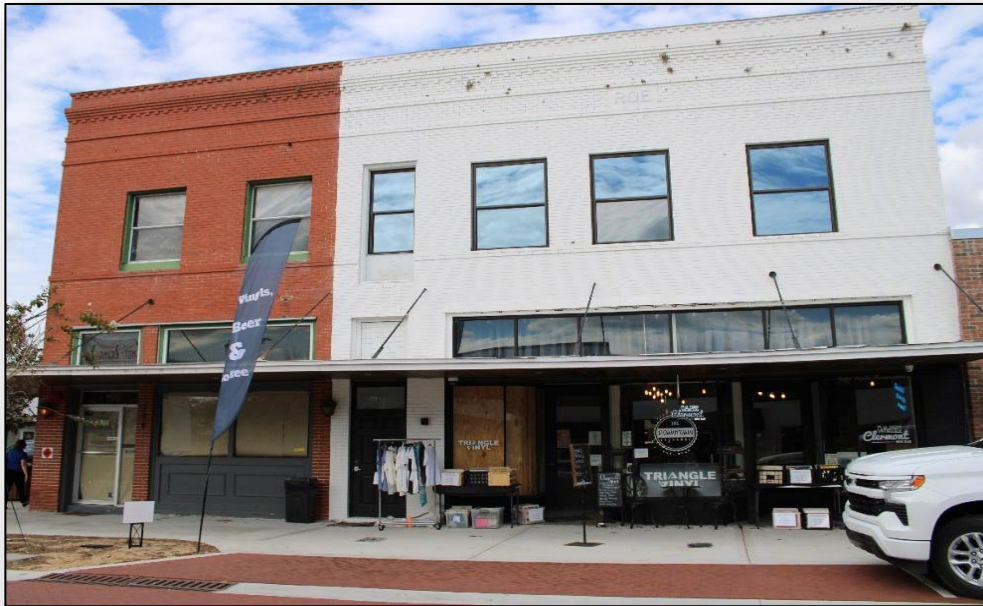
Figure 82 – 792 W. Montrose Street (LA05602) Two-Part Commercial
