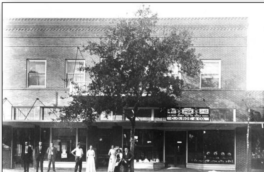
Figure 25 – Roe Building, 798 W. Montrose Street (LA05604), built in 1912.
