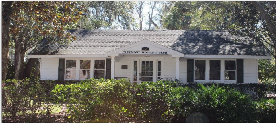
Figure 87 – 655 W. Broome Street (LA00533) Colonial Revival
