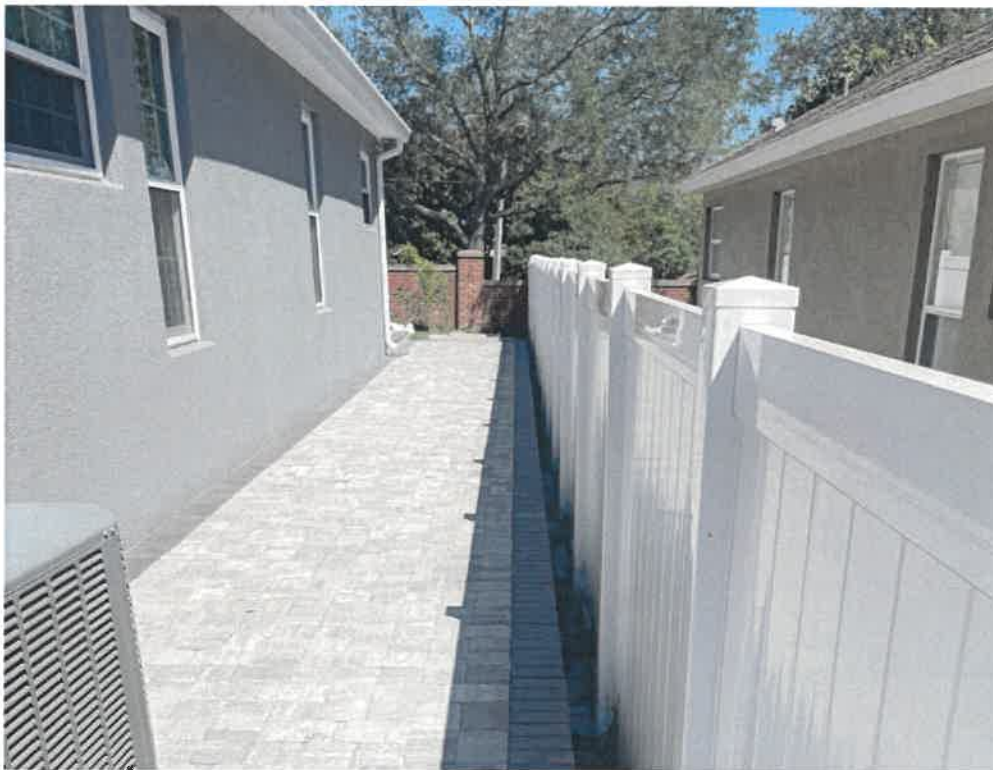
Figure 5 – South Property Line
