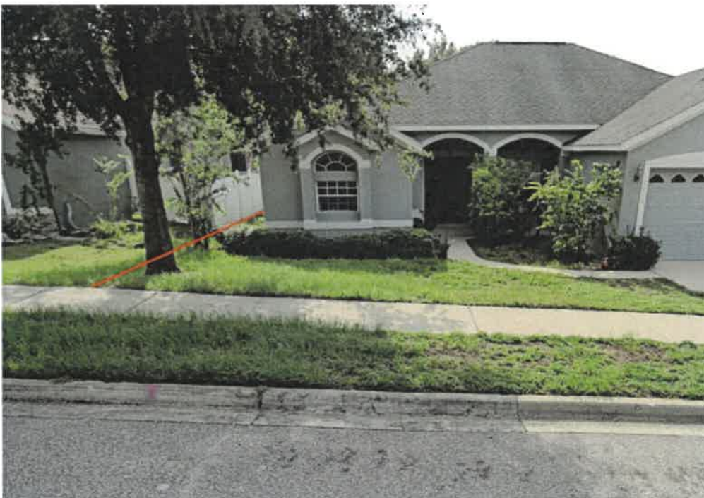
Figure 2: North Property Line Before Pavers
