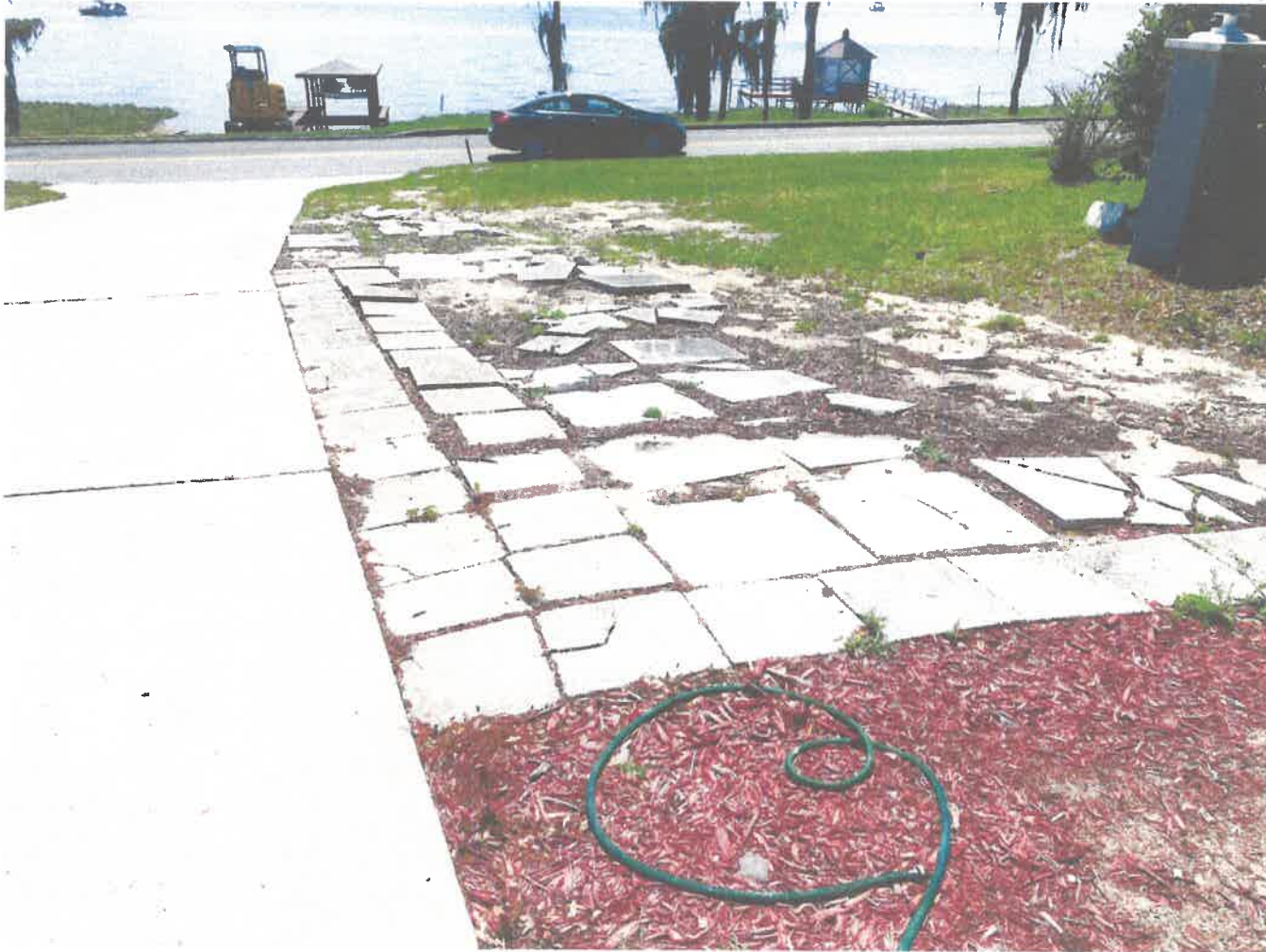
Existing Pavers on Property when Purchased
