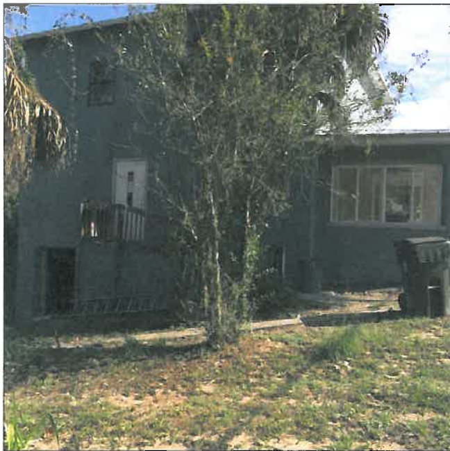
PHOTO # 4 WEST ELEV., LOOKING AT RAMP TO 2nd FLOOR LEVEL
