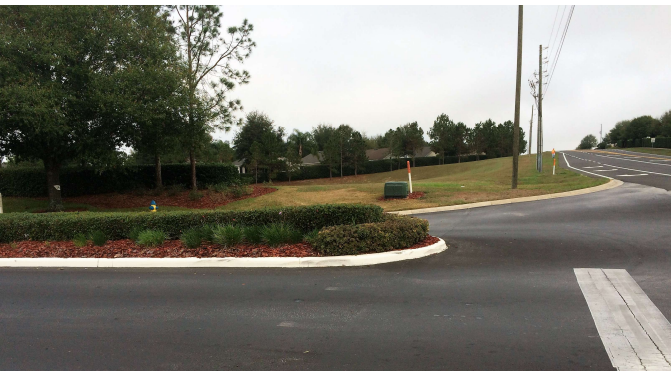
Kings Ridge Blvd, looking north at S. Hancock Road
