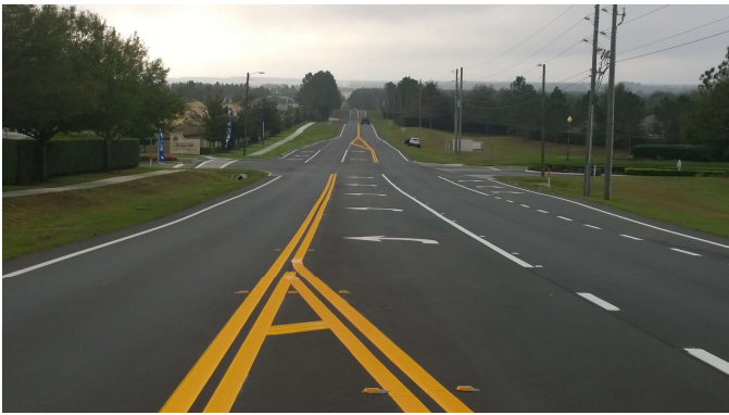
S. Hancock St SB at Kings Ridge Blvd.
