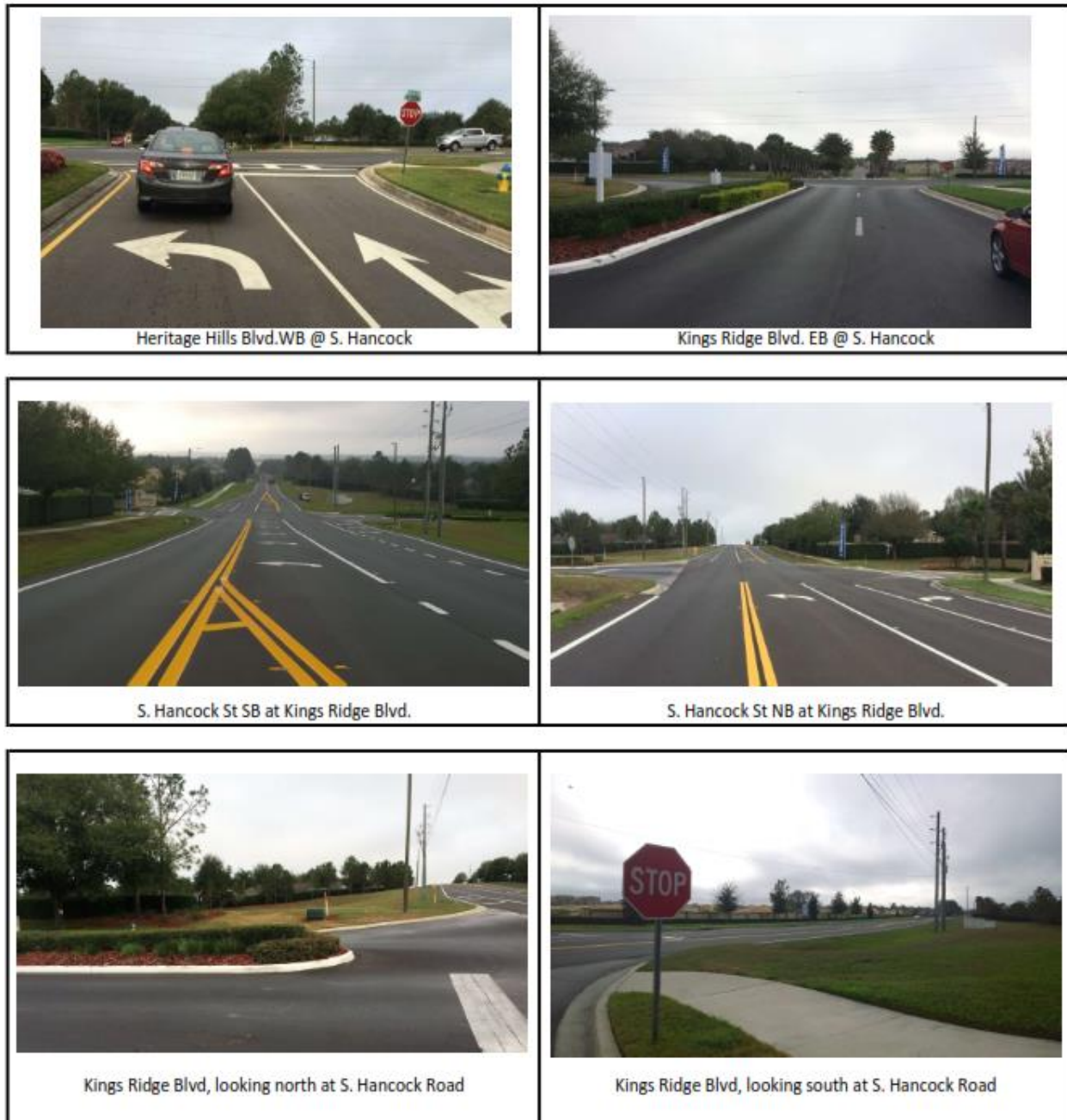
Figure 4 Photos of existing conditions at S. Hancock Road and Kings Ridge Boulevard / Heritage Hills Boulevard
