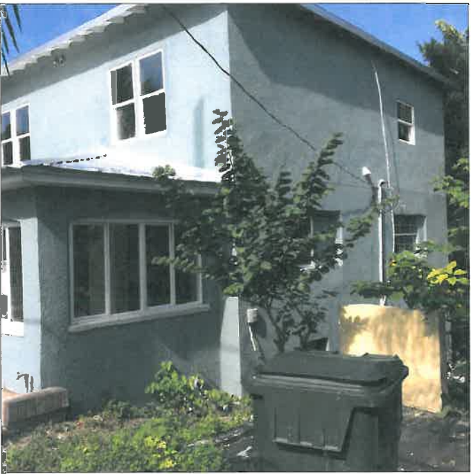
PHOTO # 6 EAST ELEV., LOOKING AT S.E. OF BUILDING
