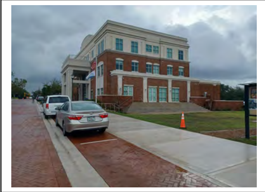
View at front of building
