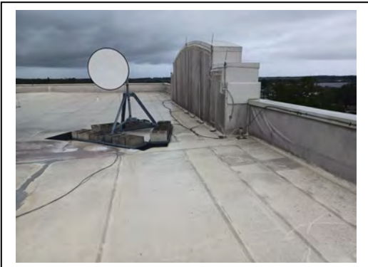
View at front parapet wall, flashing and coping condition
