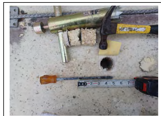
View of core sample high point behind front parapet wall
