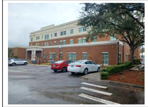
View at rear of building
