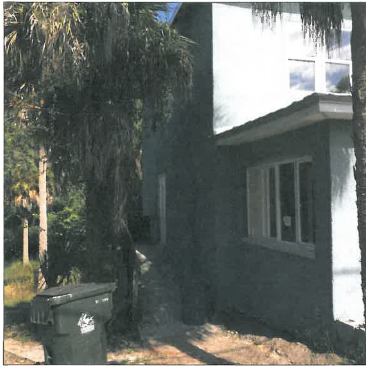
PHOTO # 1 WEST ELEV., LOOKING AT RAMP TO 2nd FLOOR LEVEL
