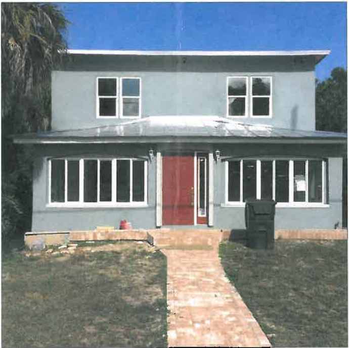
PHOTO # 5 SOUTH ELEV., LOOKING AT FRONT OF BUILDING
