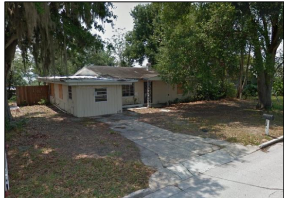
Cracked Driveway & boarded up windows
