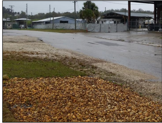
Sand & gravel driveways overflowing into right-of-way
