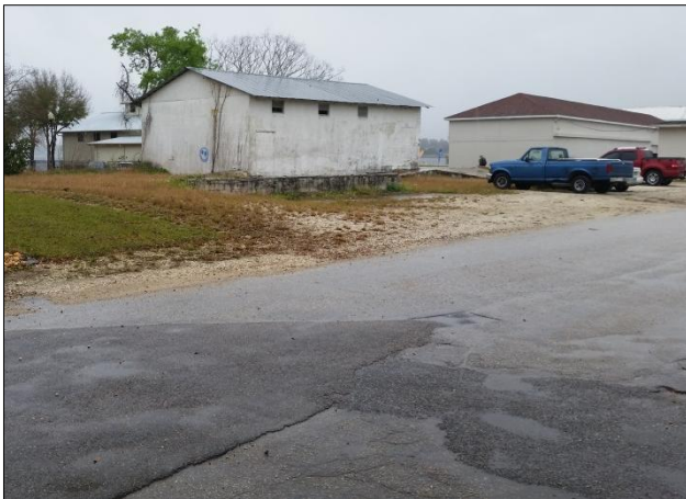
Deteriorated road, lack of curb, gutter & sidewalk
