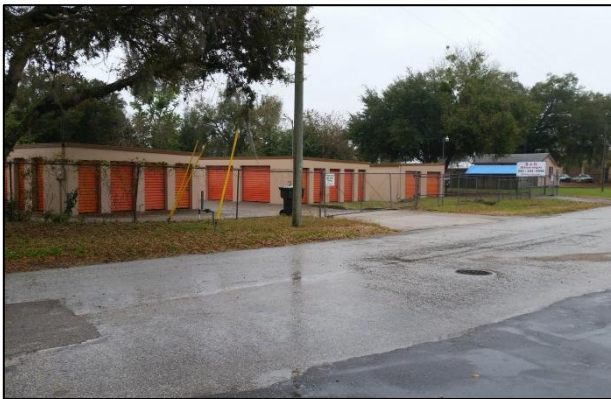
No sidewalks, curbs or gutters
