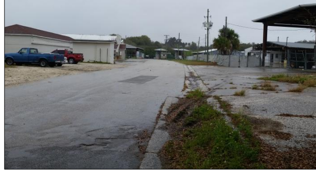
Cracked overgrown driveways & dirt driveways
