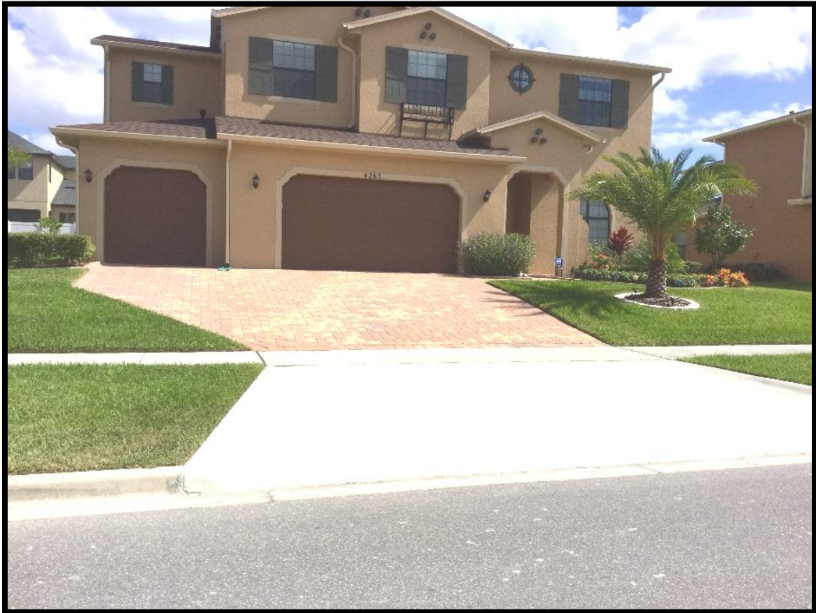
City of Clermont - Existing Three Vehicle Garage Driveway Example
