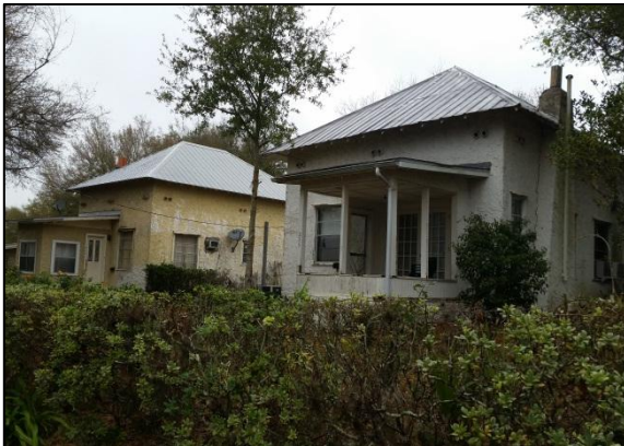
Neglected structures & overgrown landscaping
