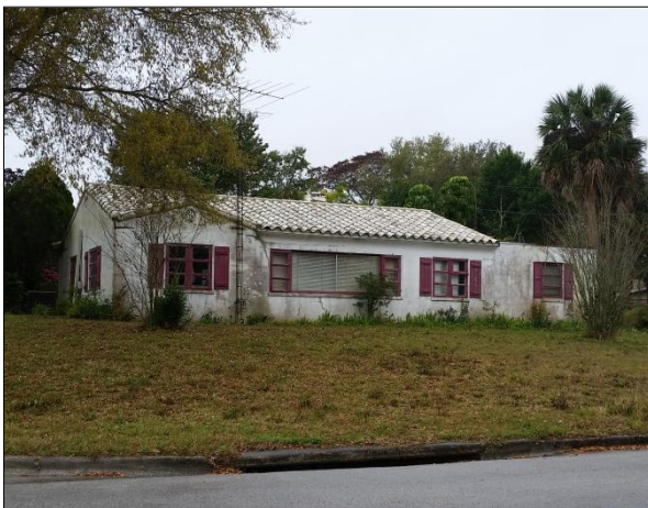
Deteriorating single-family structure
