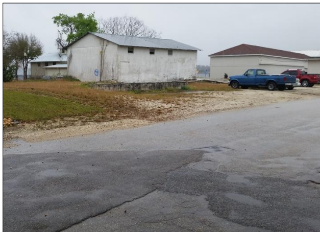
Deteriorated road, lack of curb, gutter & sidewalk
