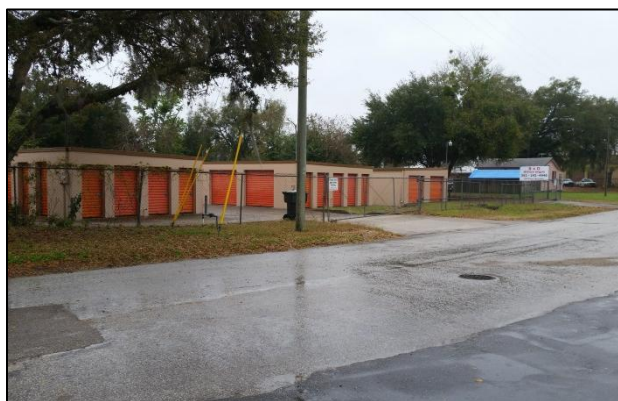
No sidewalks, curbs or gutters
