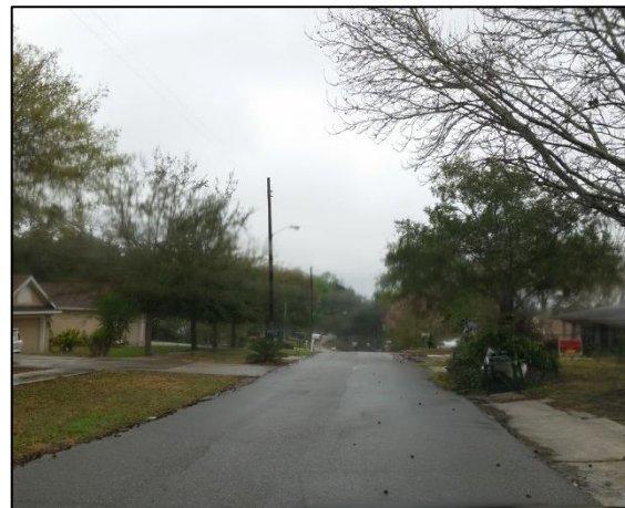
Sidewalk on one side only; missing curb & gutter
