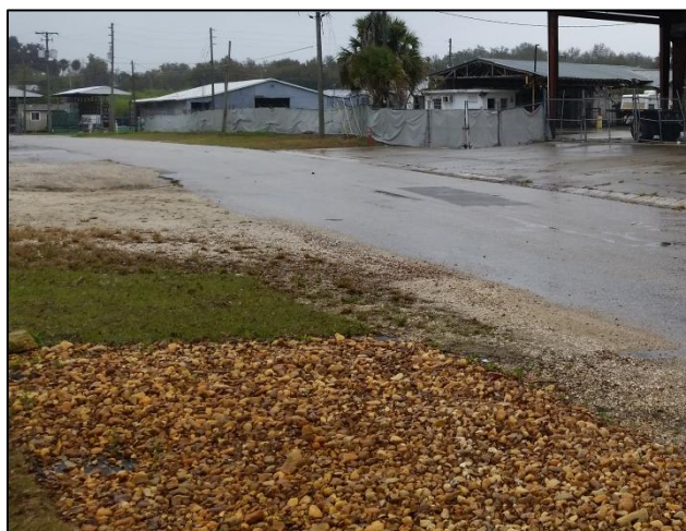
Sand & gravel driveways overflowing into right-of-way
