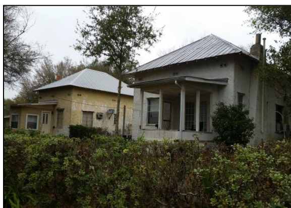
Neglected structures & overgrown landscaping
