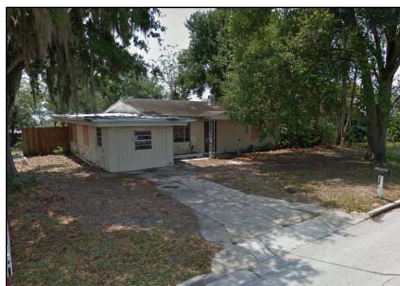
Cracked Driveway & boarded up windows
