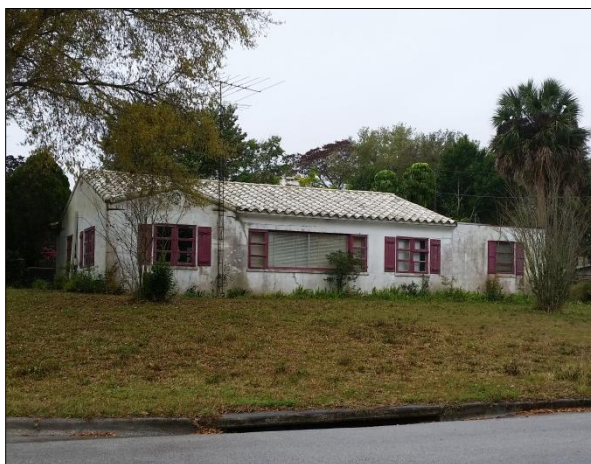
Deteriorating single-family structure
