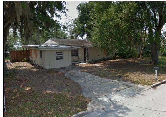
Cracked Driveway & boarded up windows
