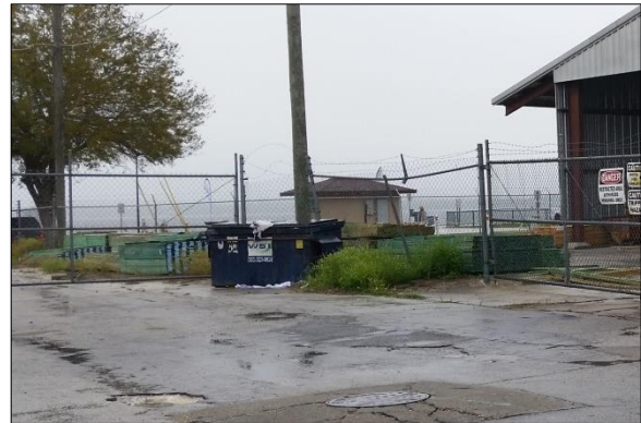
overflowing dumpster within right-of-way
