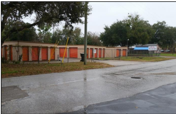
No sidewalks, curbs or gutters
