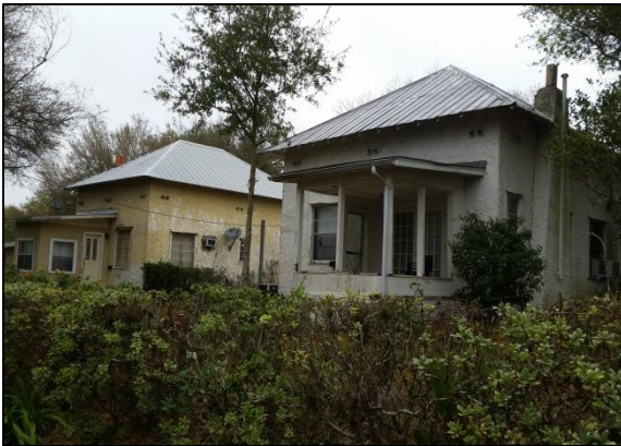
Neglected structures & overgrown landscaping
