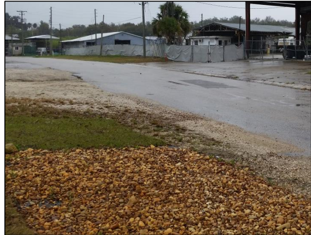
Sand & gravel driveways overflowing into right-of-way
