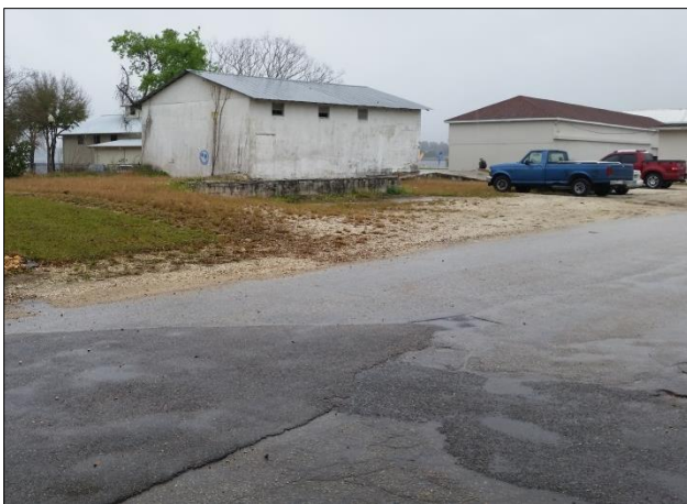
Deteriorated road, lack of curb, gutter & sidewalk
