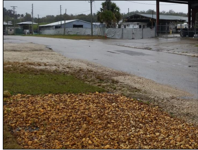
Sand & gravel driveways overflowing into right-of-way
