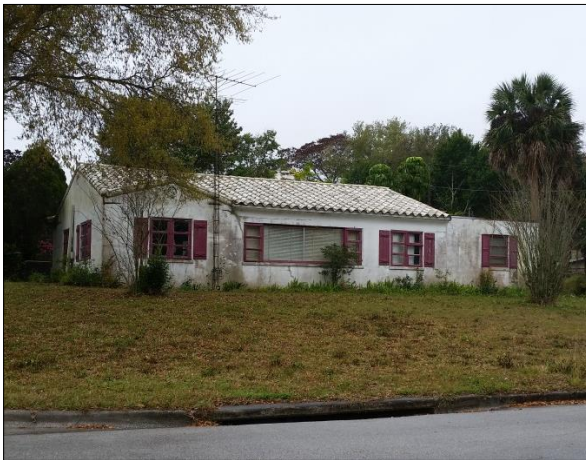
Deteriorating single-family structure
