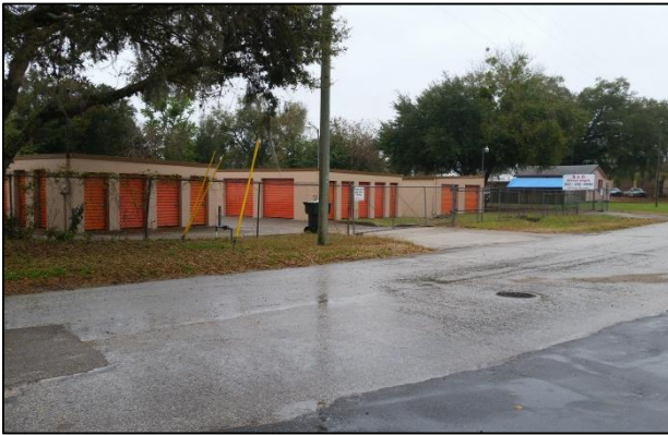
No sidewalks, curbs or gutters
