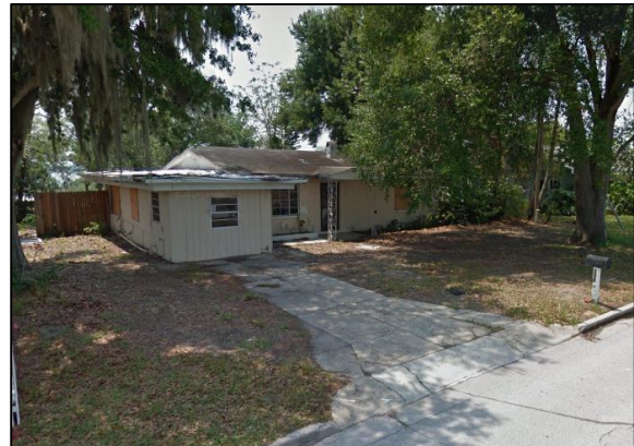
Cracked Driveway & boarded up windows
