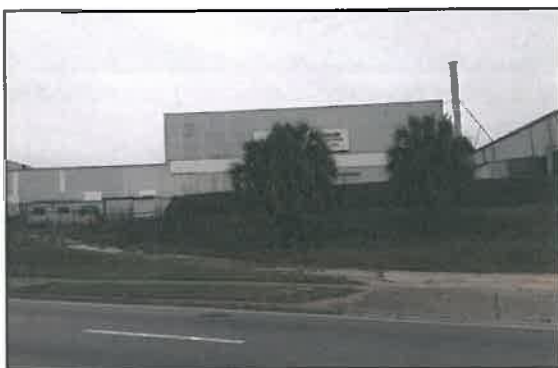
Overgrown landscaping & cracked pavement
