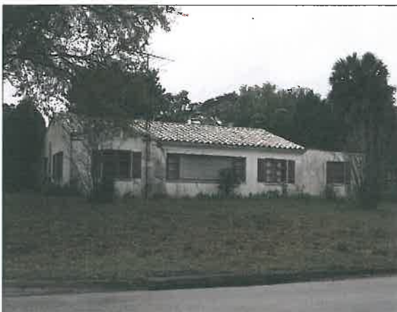
Deteriorating single-family structure
