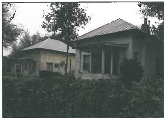
Neglected structures & overgrown landscaping
