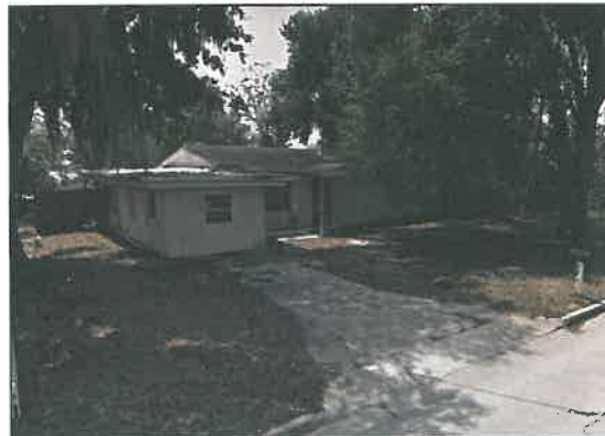
Cracked Driveway & boarded up windows
