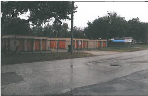
No sidewalks, curbs or gutters
