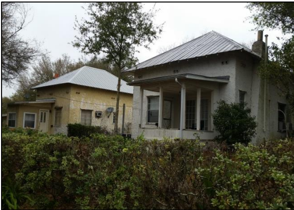
Neglected structures & overgrown landscaping
