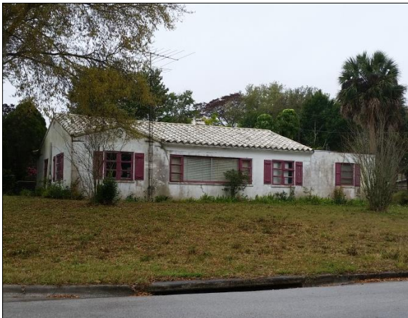
Deteriorating single-family structure
