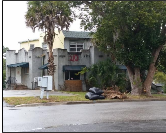
Deteriorated multi-family structure
