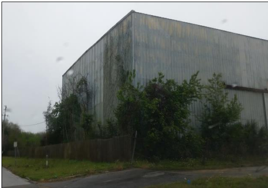
Overgrown landscaping & dilapidated fencing
