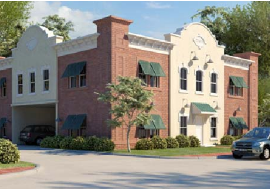
typical 2 story commercial/office building
