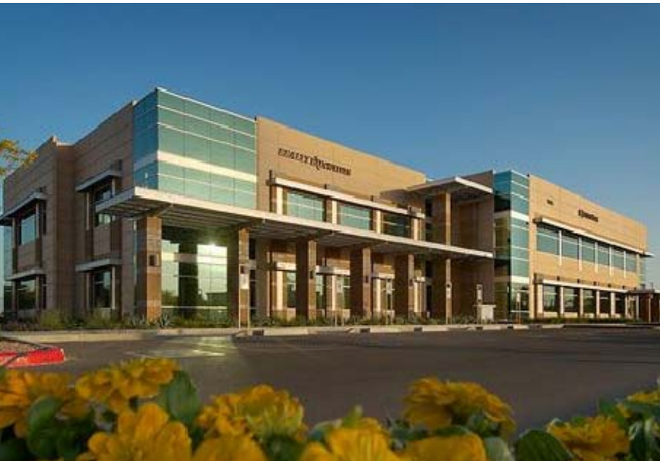
typical 2 story commercial/office building
