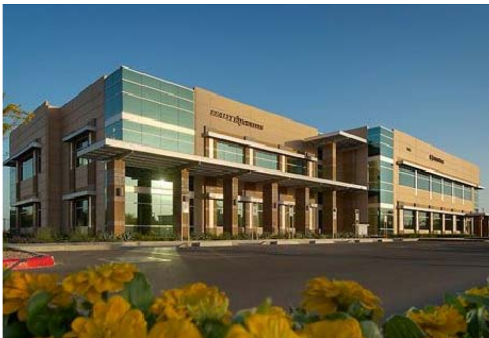
typical 2 story commercial/office building
