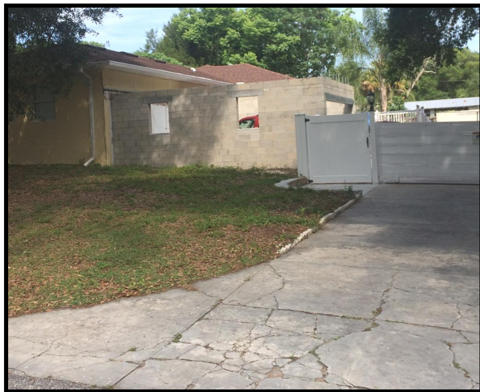
Garage that is being reconstructed
