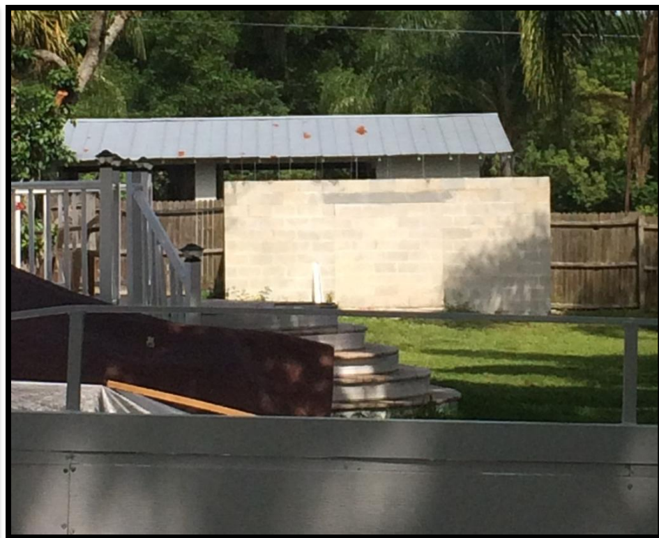
Shed that is being reconstructed
